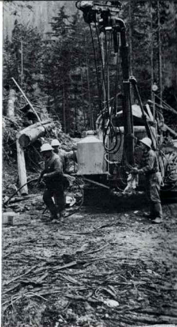
Logging in the Mamquam Valley proceeded rapidly once road building difficulties were overcome. Right: Road builders blow blasting agent into bore hole before moving drill rig safe distance from blast.
