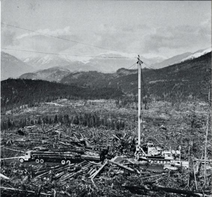
Logging in the Mamquam Valley proceeded rapidly once road building difficulties were overcome. Right: Road builders blow blasting agent into bore hole before moving drill rig safe distance from blast.
