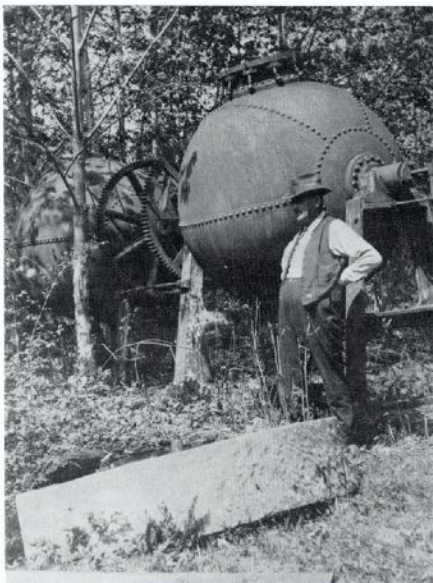
Original digesters installed in B.C.'s first paper mill at Port Alberni.
