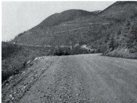
Well graded wide logging roads to upper levels made possible with modern road building equipment have assisted in logging of higher areas.
