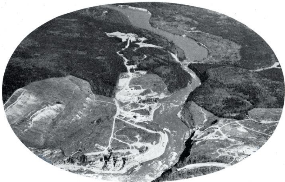
Overall view of Peace River Power Project under development by the B.C. Government. Dam will extend across cleared areas in bottom part of picture.
