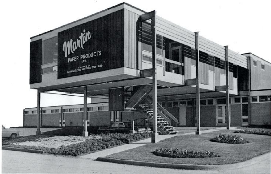
New Winnipeg Plant for Martin Paper will be similar in design to Calgary plant (above) opened last year.
