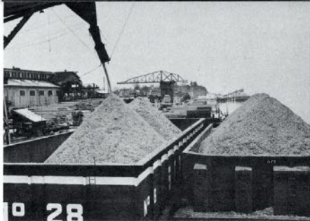
Installation of chippers in sawmills has allowed former waste slabs, edgings, etc., to be chipped for pulp. Chips being loaded at our Chemainus sawmill for our Harmac pulp plant.
