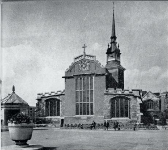
All Hallows by the Tower restored. Original stone work can be seen in the two wings and across bottom center.
