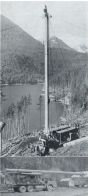
Portable spar quickly erected and in operation. Inset: in portable position for move to new site.
