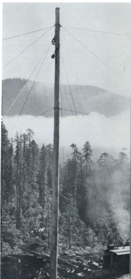
Rigging a stationary spar tree took several days.
