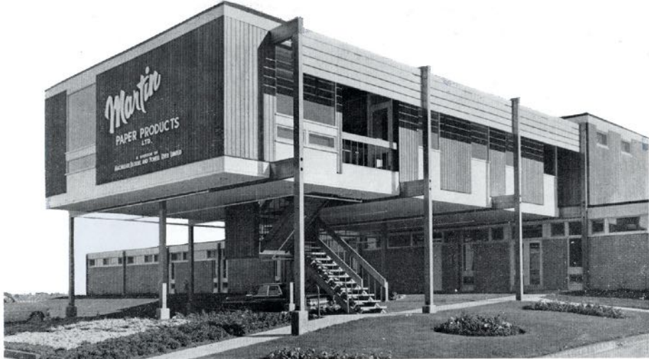
Front of new plant showing office section with service wing extending across ground level.
