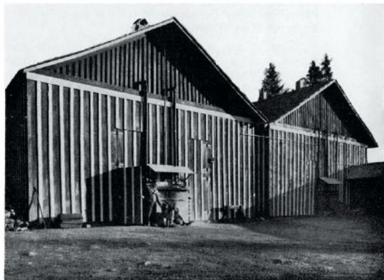
Two of Mr. Papke's five mushroom houses, each containing several beds.
