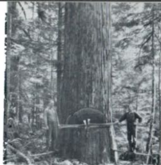
The old method of hand falling—a long and tedious job.
