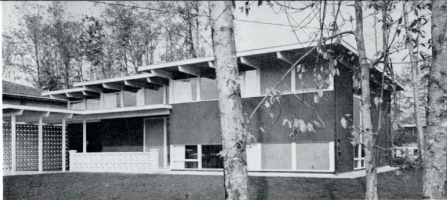
An attractive design is created by using different types of Sylvaply. Here Channelply and Smooth-face are combined.
