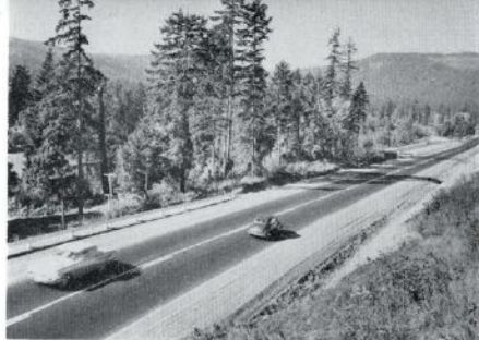
Typical Vancouver Island highway.
