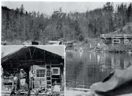
Former Hudson's Bay warehouse at Laketon is now used as a summer camp. Inset, owner on front porch of building.
