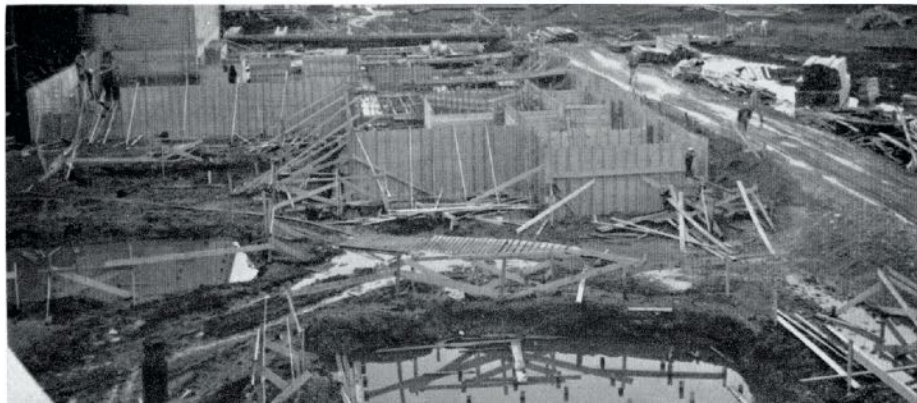
Start of construction on new newsprint machine project at Port Alberni.
