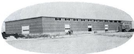
Saskatoon Warehouse nearing completion.
