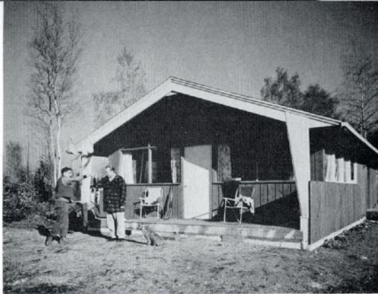
The rigid frame building system lends itself ideally to summer homes because it is so easy for amateur builders to erect.
