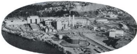
Port Alberni Pulp and Paper Plant.
