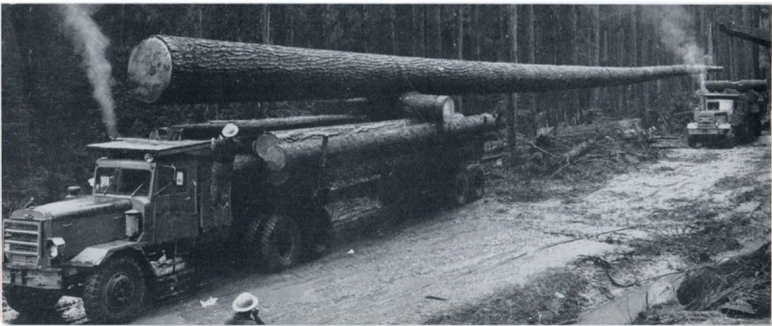
225' pole from Copper Canyon was transported by two logging trucks.
