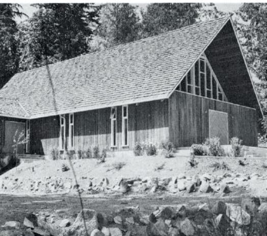
St. Matthew's Church, Horseshoe Bay, B.C., roofed with heavy resawn handsplit cedar shakes.
