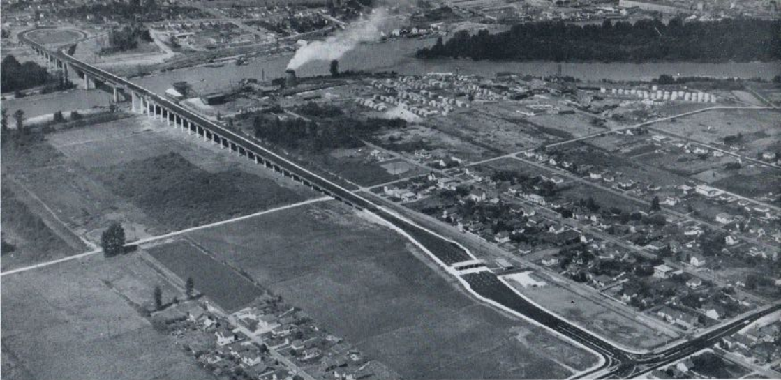
New Queensborough Bridge across Fraser River at New Westminster.
