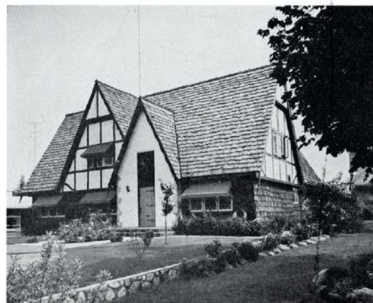
Residence in Vancouver, B.C. Tapersplit red cedar shakes on roof and sidewall.
