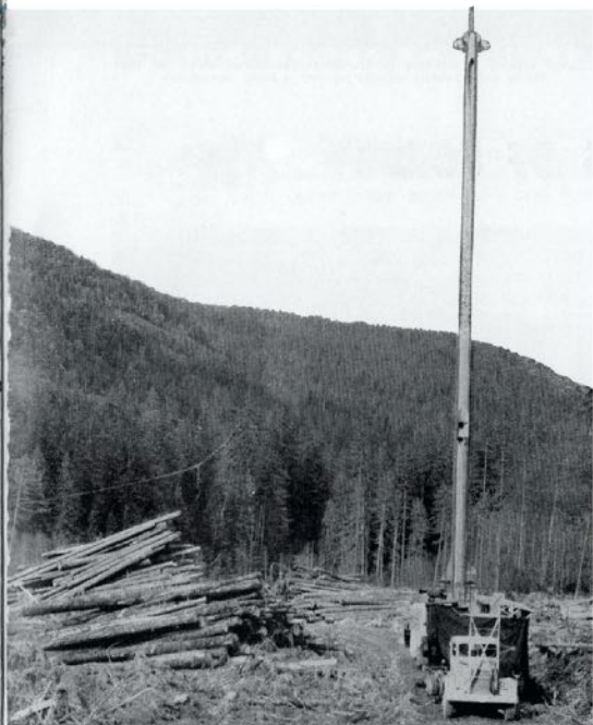
Portable steel spar, latest acquisition in western logging, yards logs ready for loading on trucks. This spar is now being used extensively in MacMillan, Bloedel and Powell River camps.
