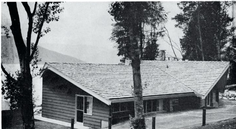
Private residence near Vancouver. It is roofed with 24" topsplit handsplit shakes in combination with cedar siding on sidewalls.
