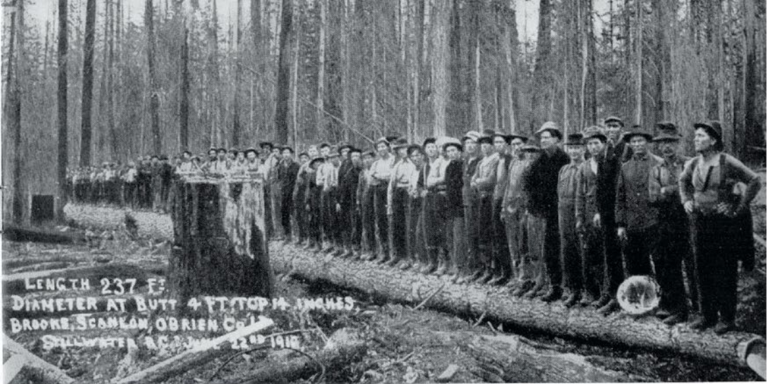
Logging crews line up on 237' pole which was erected at Kew Gardens in 1919.
