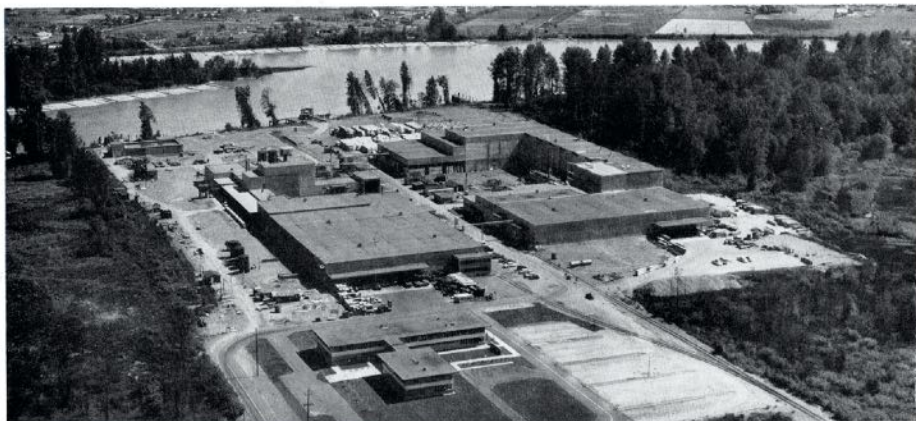
Sidney Roofing & Paper Company plant in Vancouver area.
