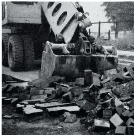
Blocks being removed show no signs of wear.
