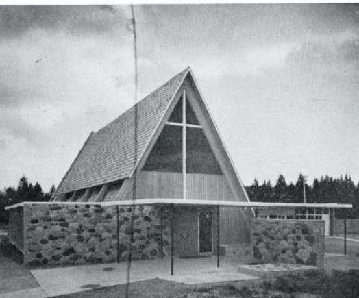
St. Anselm's Church, Vancouver, B.C., roofed with handsplit and resawn red cedar shakes.
