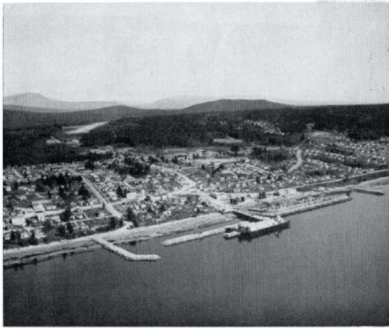
Small boat harbour at Westview extends out both sides of Government wharf. New area on left of wharf.
