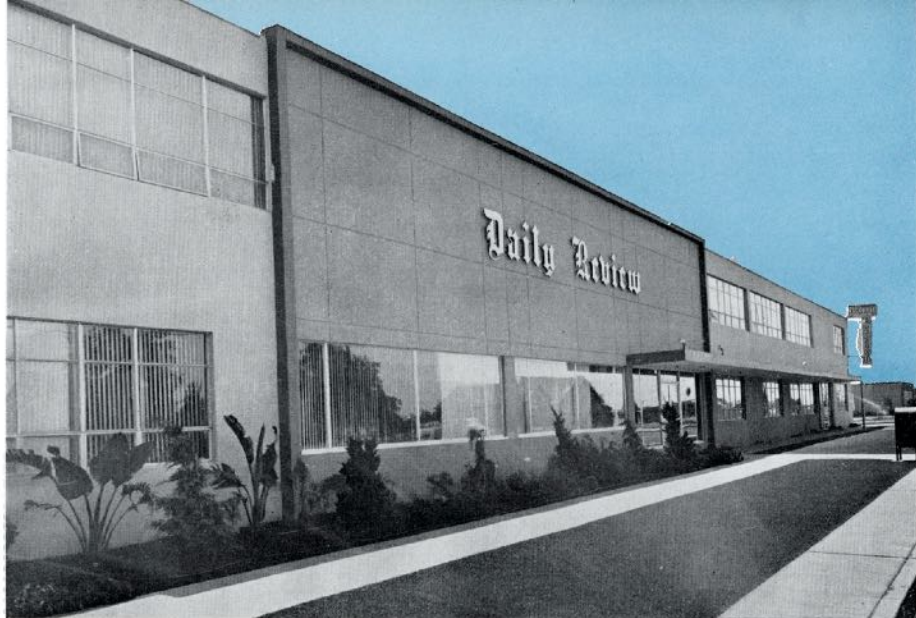
The new Daily and Sunday Review building sits on 3½ acres at 116 W. Winton Avenue, Hayward, Calif. Occupied in November, 1957, the plant has 33,000 square feet of working space on two floors.
