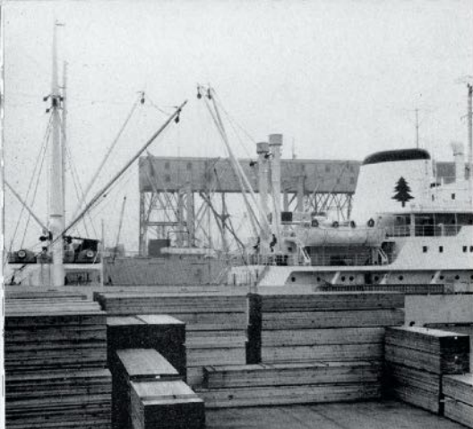
Packaged lumber at shipside, Vancouver.
