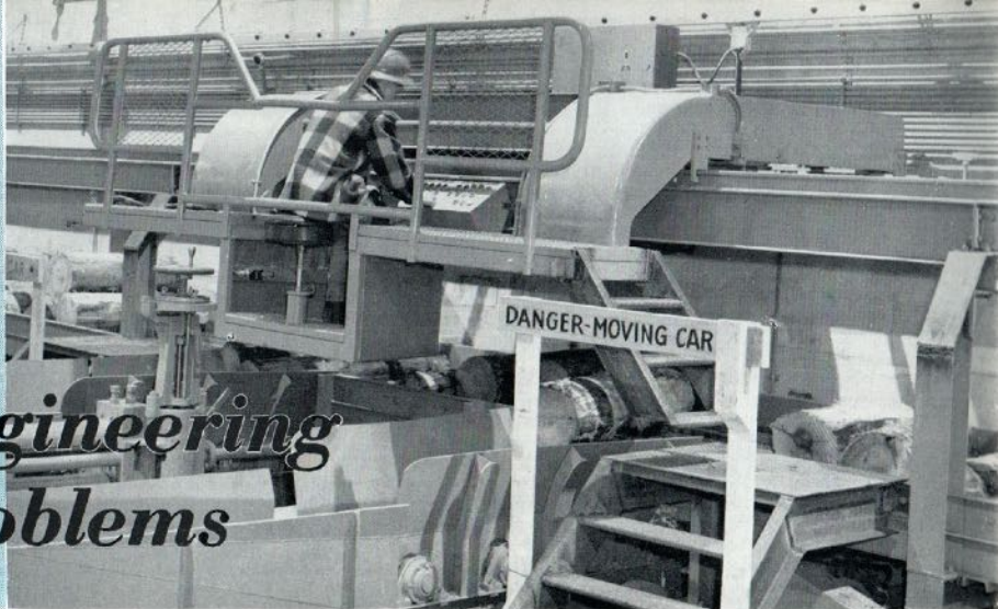
From his travelling carriage the operator can alternately feed the four grinders in the new groundwood room.
