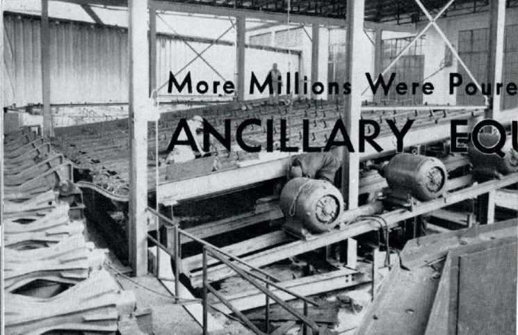
An all-metal slasher deck was among many additions required to keep Number 9 adequately supplied with logs.
