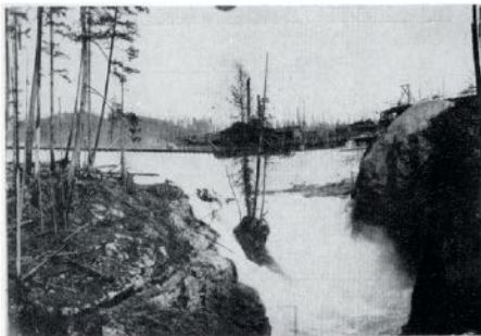
Powell River was originally chosen as the site for a paper mill because of the adequate supply of water from Powell Lake. The early (1911) dam, left, was enlarged to develop its present 50,000 h.p. An additional source of power was obtained in 1930 (see lower pictures).
