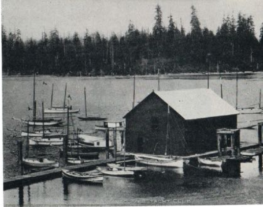
Original quarters of the R.V.Y.C. in the first decade of this century.
