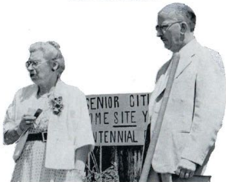
Reeve Ray Weaver and Mrs. A. Devaud officiate at ceremony beginning construction of Powell River's Senior Citizens' Home. (P.R. News photo).
