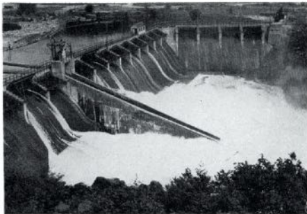
Powell River was originally chosen as the site for a paper mill because of the adequate supply of water from Powell Lake. The early (1911) dam, left, was enlarged to develop its present 50,000 h.p. An additional source of power was obtained in 1930 (see lower pictures).
