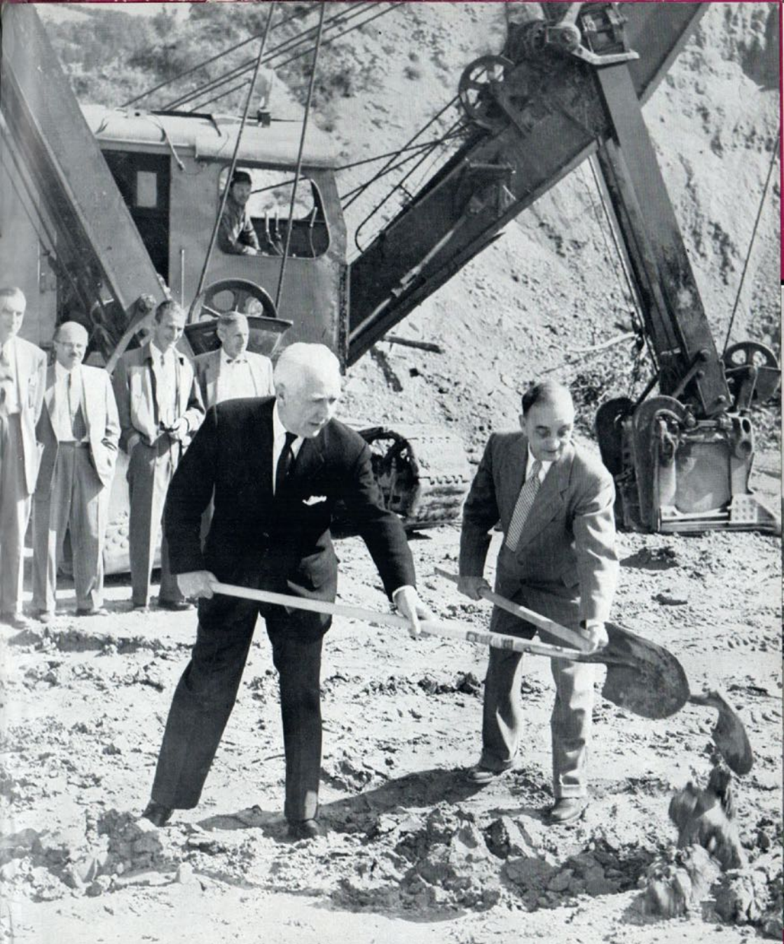
First shovelful of earth on the site of Powell River's ninth paper machine are turned over by H. S. Foley, Chairman of the Board, left, and F. C. Powell, the Company's longest service employee. Nearly $20,000,000 will be involved in Powell River's latest expansion program. (Story on page 1)
