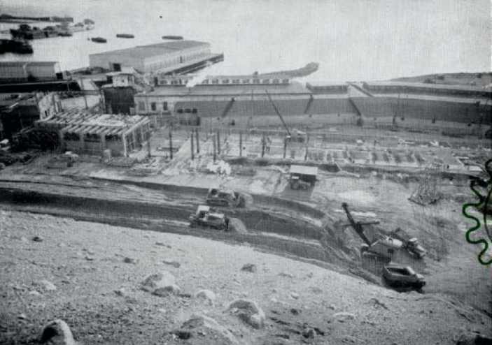
No. 9 Machine Room construction well under way.
