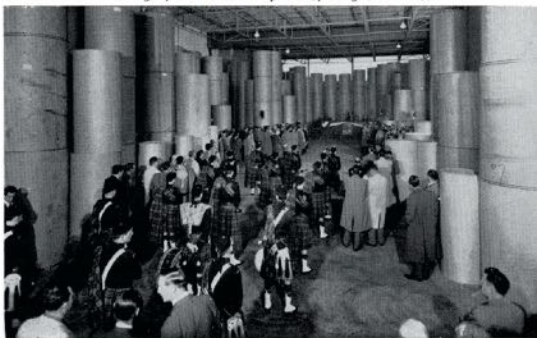
Kraft rolls in storage provided backdrop for opening ceremonies
