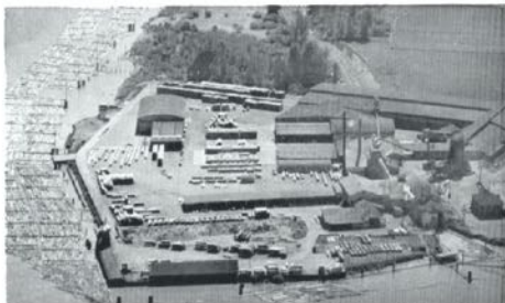
Safest sawmill in its class is the B.C.M. Plant at New Westminster
