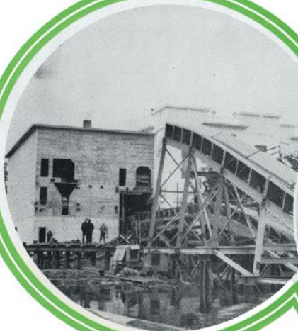
Barker Mill Addition Is Nearing Completion.
