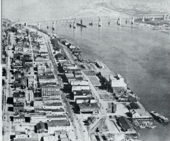
Pattullo Bridge spans the Fraser at New Westminster
