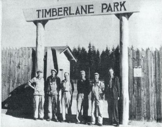
Townsite crew built this arch.
