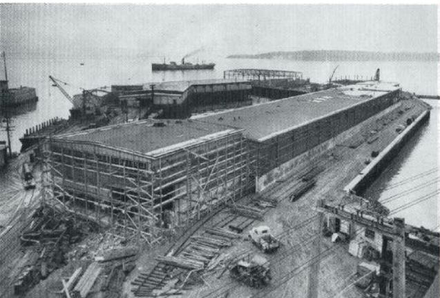
The new wharf warehouse nears completion.
