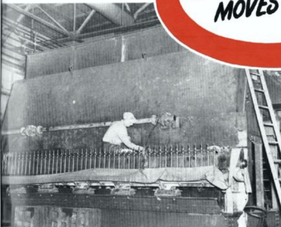
Setting in new head box on No. 5 Paper Machine.
