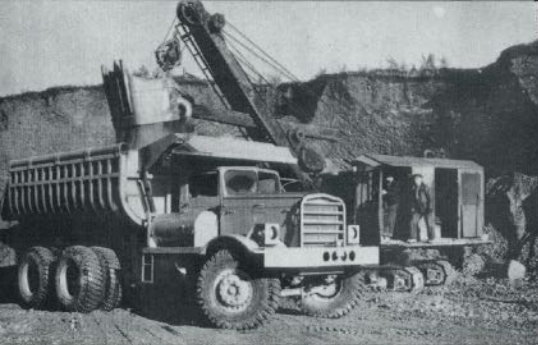
Modern Equipment Used In Road-Building
