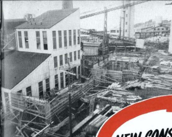
Steam plant extensions under way.
