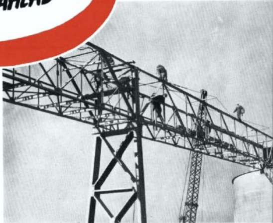
Chip conveyor system.
