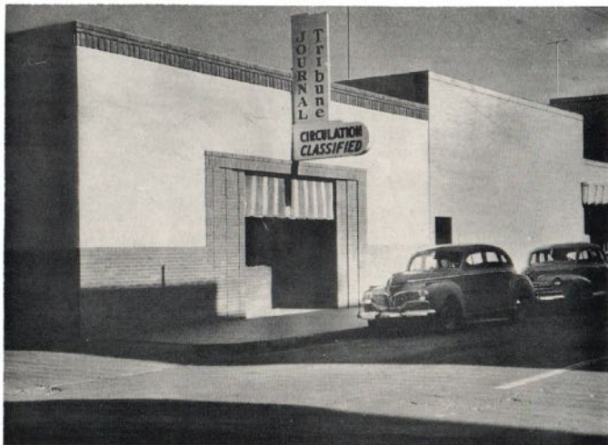
Recent addition to the plant of the Albuquerque Journal-Tribune, Albuquerque, New Mexico, houses the circulation and classified departments of one of the Southwest's most influential morning and evening newspapers.
