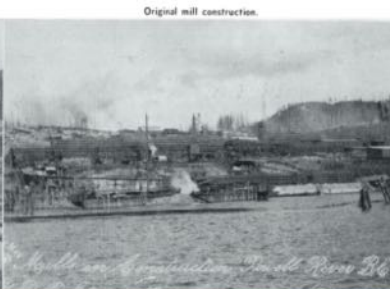
Original mill construction, 1911-1912.
