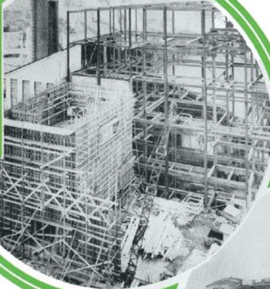
New Steam Plant Takes Shape
