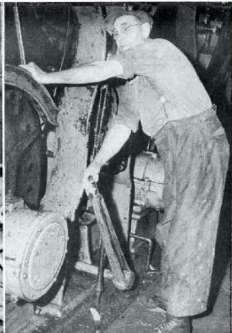
Ray Gribble shuts down dryers
