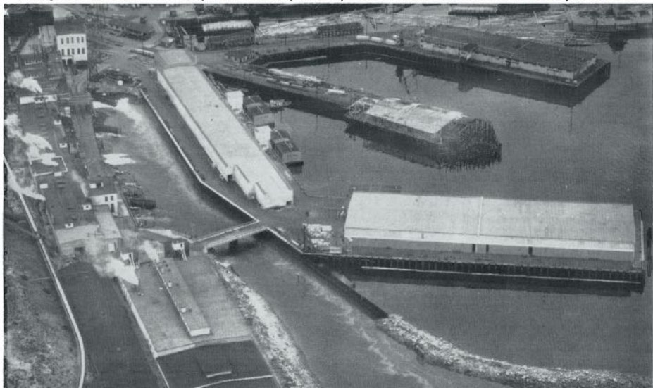
Powell River's new wharf and warehouse, showing its relation to existing installations. The old wharf in the centre, which forms part of the original structure built in 1911-1912, will be eliminated, and the space between the two outside wharves will form a protective basin.
