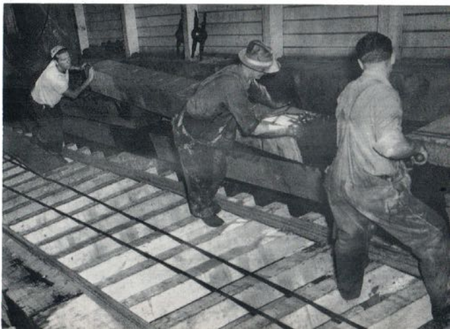
Replacing timbers on an inclined elevator.
