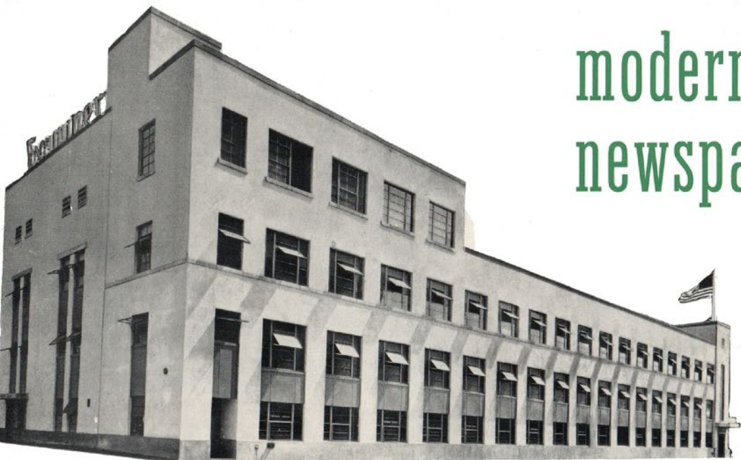
Mechanical annex of the Los Angeles Examiner, put into operation in October, 1949, houses the pressroom, stereotype, foundry and mailroom in its 88,000 square feet of floor space.
