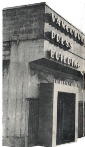
Located two blocks away from Vancouver landmark, this functioned expressly for The Vancouver S
