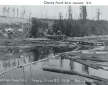
Clearing Powell River townsite, 1910.
