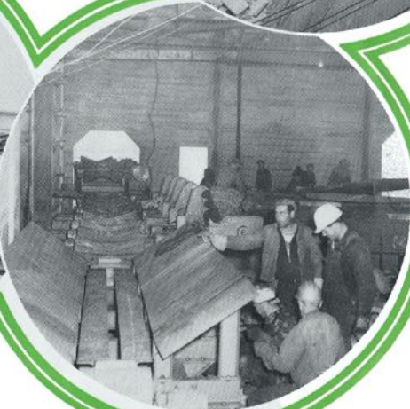
Installation of Intermediate Barker Is Well Under Way.
