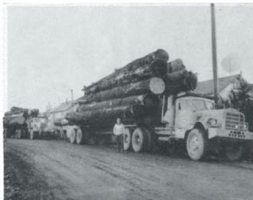
Roads Must Be Built To Withstand Heavy Loads. Front Truck Carries 90,000 Lbs.
