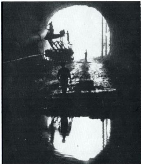
Diversion Tunnel, Nechako Canyon Damsite.
