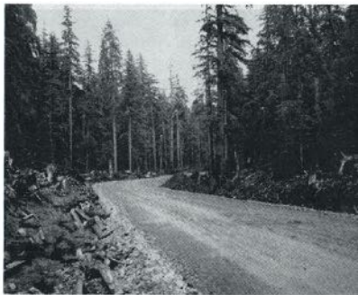
Type of two-way gravelled highway at Juskatla, capable of handling 100 ton loads.
