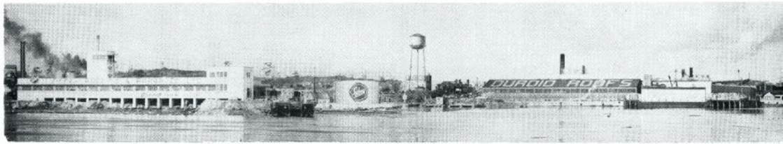
View of Victoria plant.
