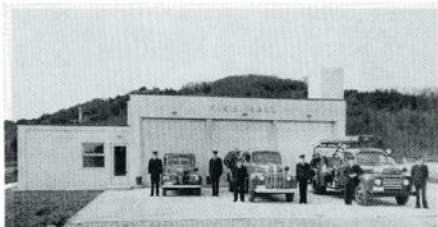
Entrance to fire hall, with permanent staff of drivers and two modern trucks.
