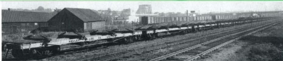
Special log cars purchased by Kelley Logging Co., Ltd., to transport pulp logs from Cariboo district to Squamish, Howe Sound.
