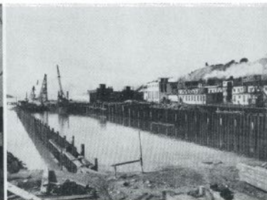
The new wharf is beginning to take shape.
