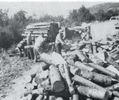
Buzz saw cuts up 8-foot sticks, hauled from the clearing operations.
