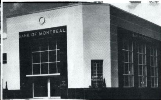
Bank of Montreal, Drive-In Branch, Vancouver, B.C.
