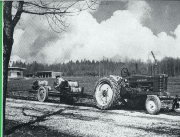
Loading bales of 2-year-old Douglas fir seedlings at Green Timbers Nursery. In last ten years Service has planted 94,000 acres of burned over forest land. To left can be seen one corner of new Ranger School Building.
