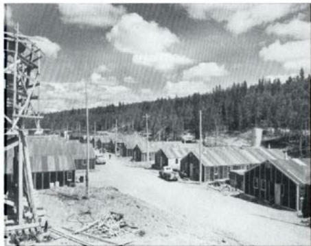
Construction Camp, Nechako Canyon Damsite.
