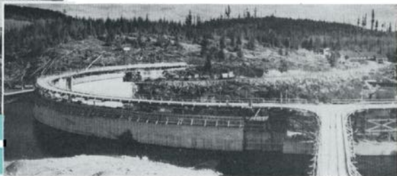
New construction will raise Scanlon Dam 20 feet.
