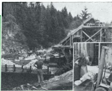
2. Dumping lime rock on scow for immediate transportation to Powell River.
