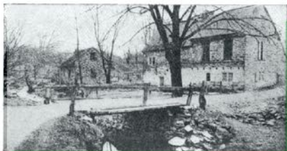
The third Rittenhouse Paper Mill, built prior to 1770.
