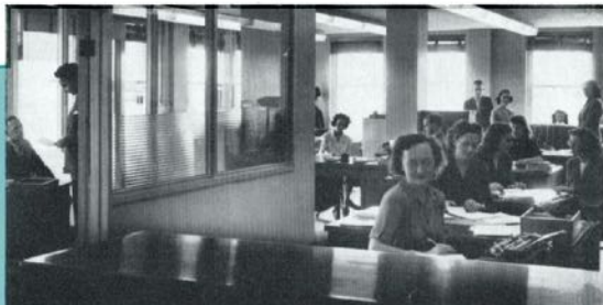
General view of purchasing office.
