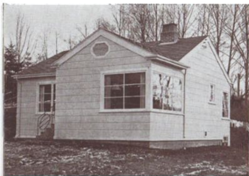
Ready for occupancy, with all fittings in.
