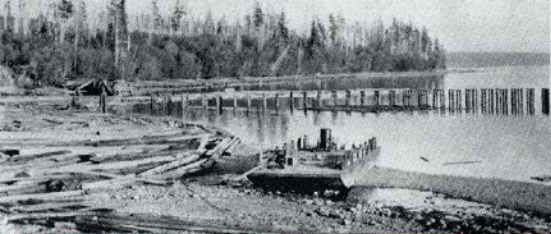
1910. Landing the pile-driving donkey from a scow at the present location of the company wharf.
