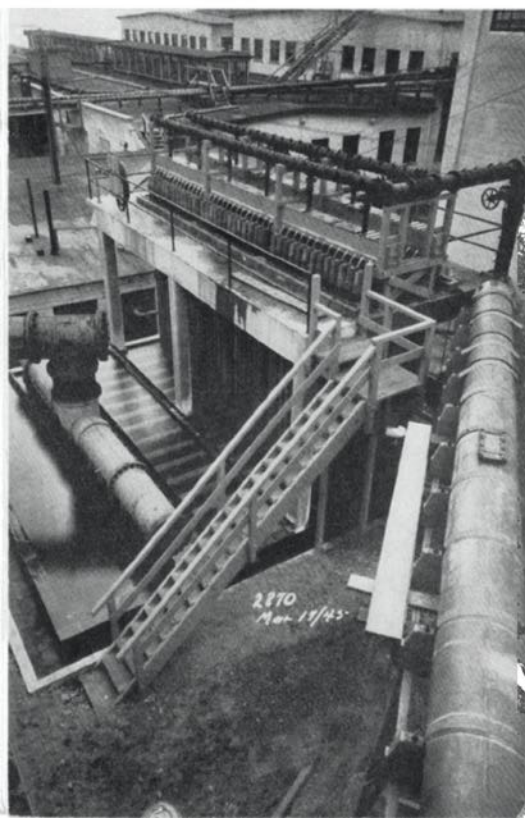
Another view of the cooler.
