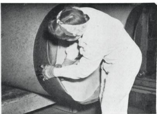
No. 4—The bands are again crimped over the edges. Seven thicknesses now protect the vital edges.
