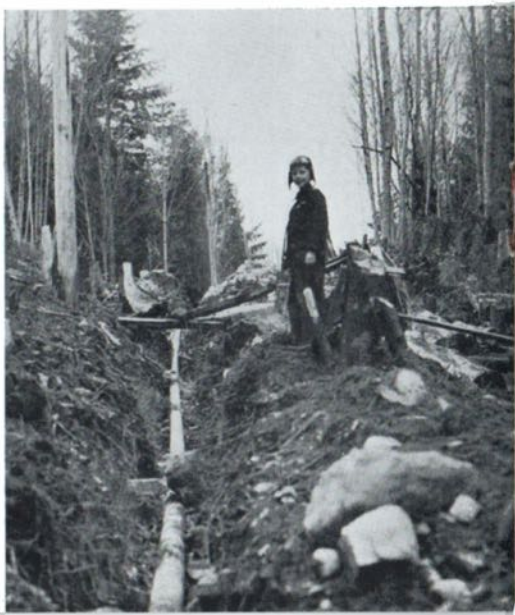
The 6-inch main line climbs 300 feet from lake level to tank 2600 feet away. It's tough country.
