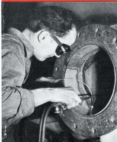
Bill Sweeney tackles a welding job.
