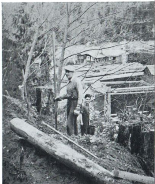
Eric Gustafson and Vito Massullo dig the pole-line bores which run to the pump site at One Mile Bay.
