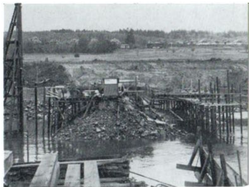
New wharf piling is shown on left beside old dismantled structure.
