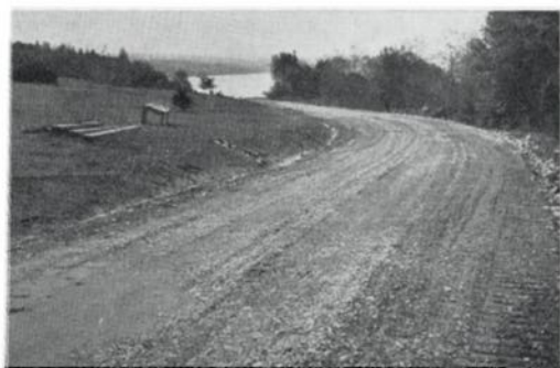
A preliminary phase of construction. New logbaul road skirting golf course.
