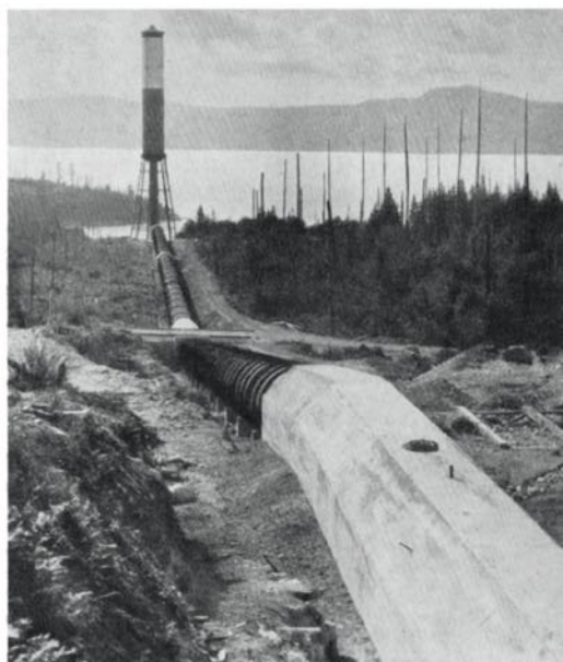
Surge tank and penstock at Lois River, where 24,000 horsepower is developed.
