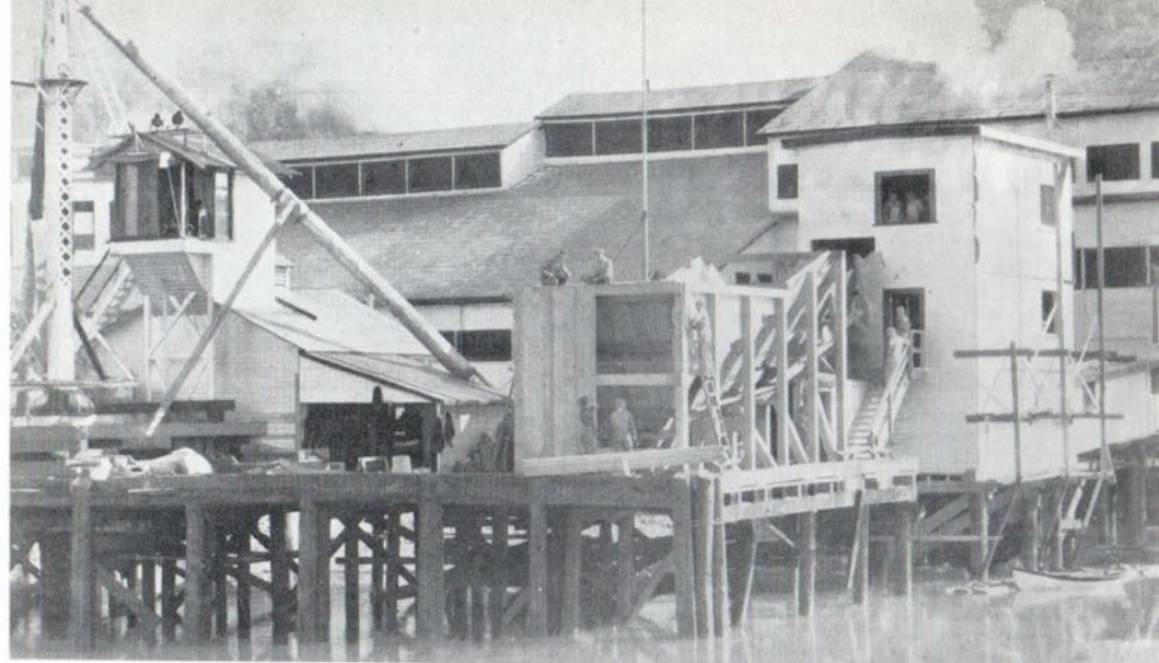
Crews put finishing touches to new machinery and building for the supply and delivery of sawmill refuse.
