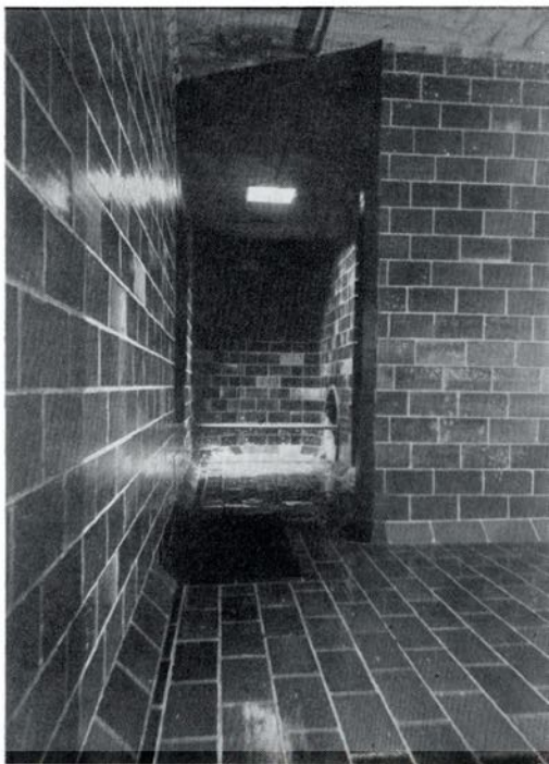
Top: Another view of the blow chest, showing the three agitators which mix the pulp. The blow nozzles from the digesters are seen in the walls. Above: The end channel and blow channel. On the left is the glazed tile lining; on the right the special brick tile installed by Stebbins. Below: Another view of one of the blow chest passages.
