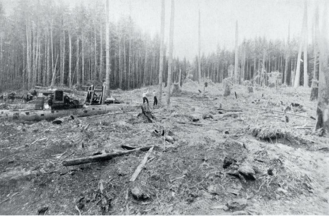
Above cut shows the setting up of equipment for the fuel cutting contract. Delivery of wood fuel will be made to Vancouver early in August.
