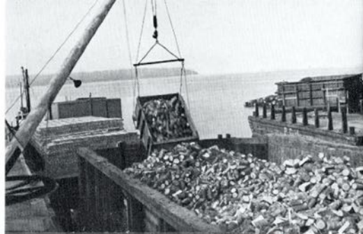
Left: Crane dumping a load of fuel wood aboard a waiting scow at Powell River. Right: Wood for Vancouver industry, a scow load of bush fuel cut from Powell River Company property.
