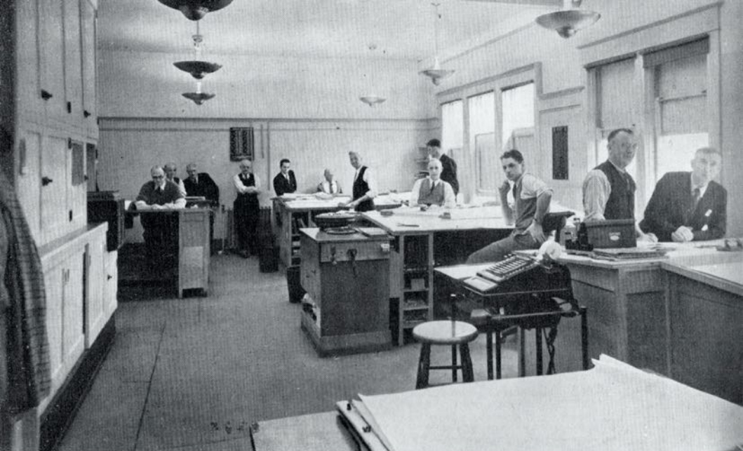
The Engineering Department Draughting Office, co-partner of the plant operating staffs. In the above picture Resident Engineer Harold Moorhead stands in the right background and Plant Engineer Archie Robertson second from left in left background. Right foreground is Wm. Jamieson, Field Engineer.
