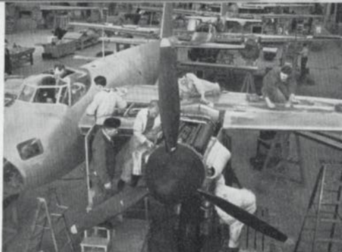
Above shows the Mosquito before and during construction. Left: the loads of big-grade spruce timber are ready for shipment from Powell River. Right: Shows construction of Mosquito planes in a Canadian factory.
