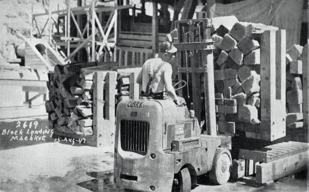
New block loading installation. The jeeps are taking a load of blocks from the pile of skips.
