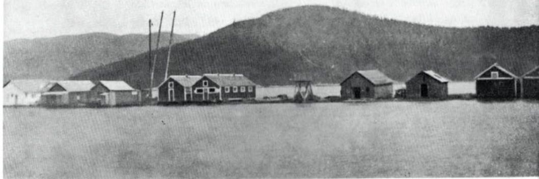
This is how they move logging camps along the B. C. coast. Bunk houses, offices, etc., are built on floats. When a move to a new camp is necessary the whole outfit, camp and machinery, is hitched together and towed away.
