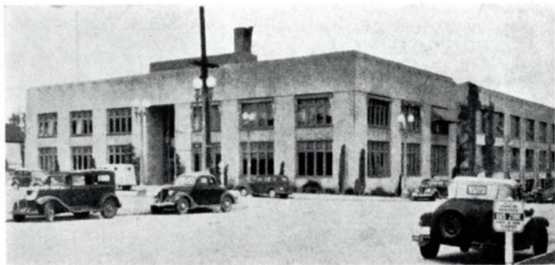
Main plant of the Seattle "Times," corner Fairview and John Streets, Seattle. The "Times" has been a steady customer of Powell River since 1914.
