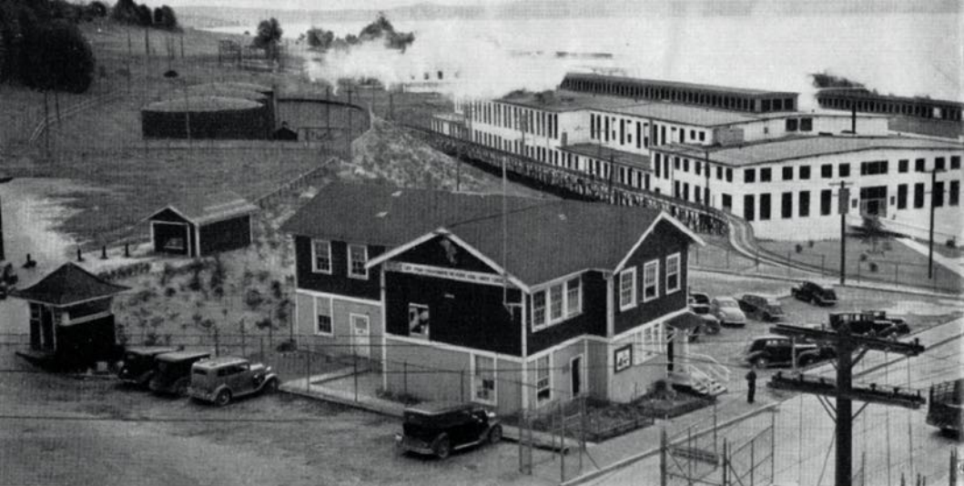
Modern view of Number 7 Machine Room buildings, with old engineering office in foreground.
