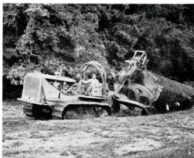
Caterpillar drawing giant spruce stick from the woods. Some of these timbers are 10 feet in diameter.
