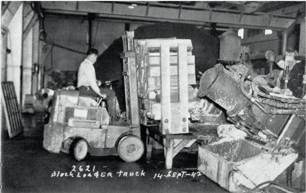
Another illustration of new method—jeeps deliver the blocks direct to the grinder machine.
