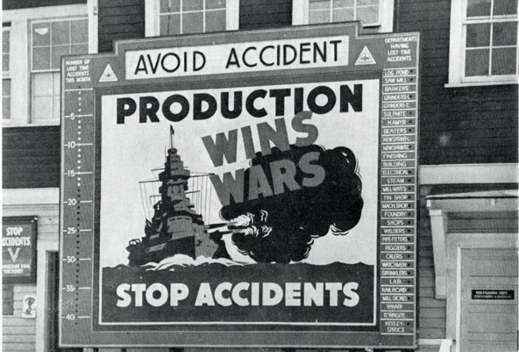
The new electric safety sign in front of the watchman's office. The big central picture is changed regularly.
