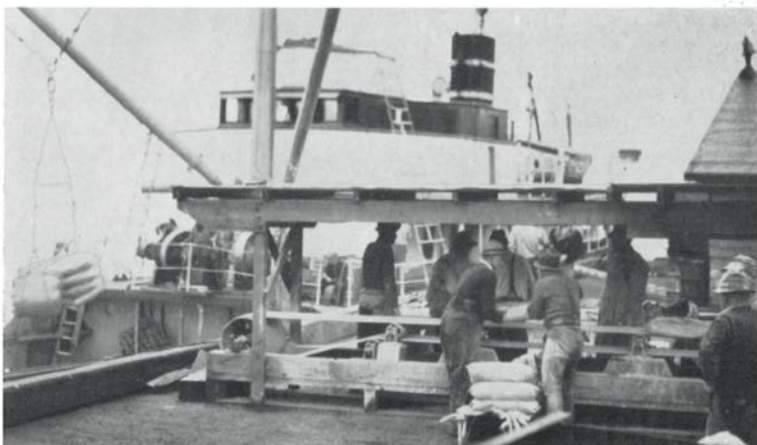
Unloading cement at Stillwater for the Lois River permanent dam. Cement is shipped direct from Vancouver and carried by logging train from Stillwater to the dam site, about two miles away.
