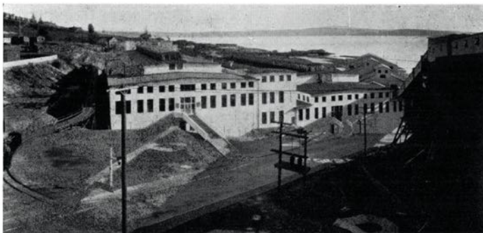
Machine room buildings at Powell River, where three of the big machines are housed. These buildings illustrate the exterior architecture of the modern machine room building.
