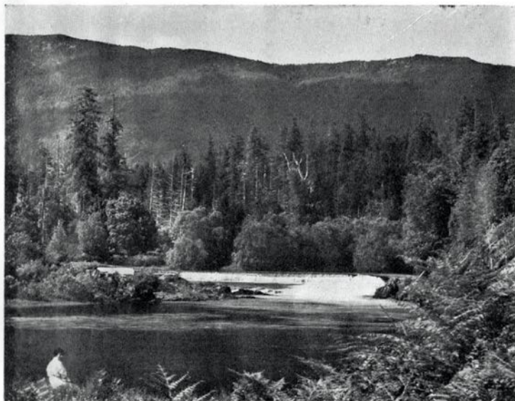
The dam of the British Columbia Paper Manufacturing Company as it appeared when the mill was in operation in 1894.
