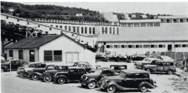
Bicycles are not of course the only transportation used by mill employees. Here are a few of the cars owned by the boys in the lower part of the plant. Several hundred cars are parked in the various plant spaces daily.
