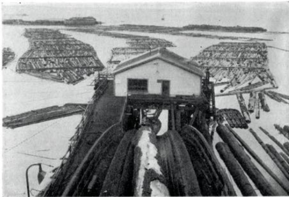
The log conveyer, showing logs on their way to the sawmill from the mill pond. In the background are seen the boomed logs awaiting their conversion to Powell River newsprint.
