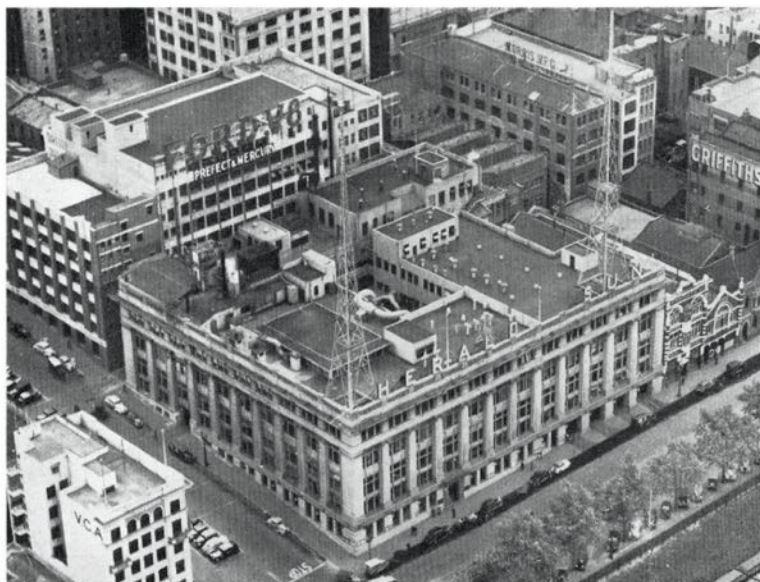
Aerial view of the "Herald-Sun" building, showing the two masts of the Herald broadcasting stations, 3 DB and 3 LK. The ventilation system can be seen in the centre of the roof. On the ground level, left hand side, is the entrance for the paper store, and the despatch dock is on the right.
