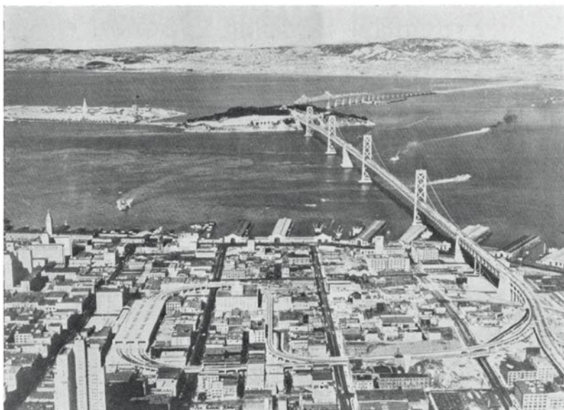
Air view of part of San Francisco Harbor, showing Bay Bridge and Treasure Island (extreme left).
