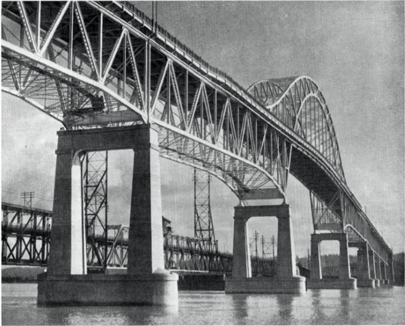
The new Pattullo Bridge, crossing the Fraser River at New Westminster. This is one of the main traffic arteries from the coast to the United States border.
