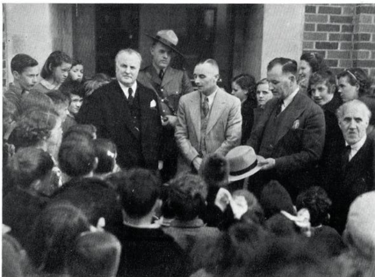
Premier Pattullo opens the new Federal Building at Powell River. Inset we show the Premier (left) with Harry Davis, President Powell River Board of Trade, and Mr. C. F. Dawson, Dominion Architect, surrounded by a group of Powell River's younger citizens.
