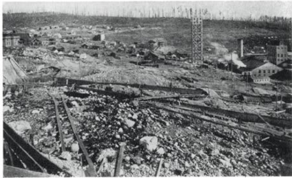
The townsite in 1911, showing beginnings of construction.
