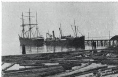
The barque "British Yeoman" bringing in the first load of concrete for plant construction in 1911. The old sailing craft were seldom seen at our dock after this date.
