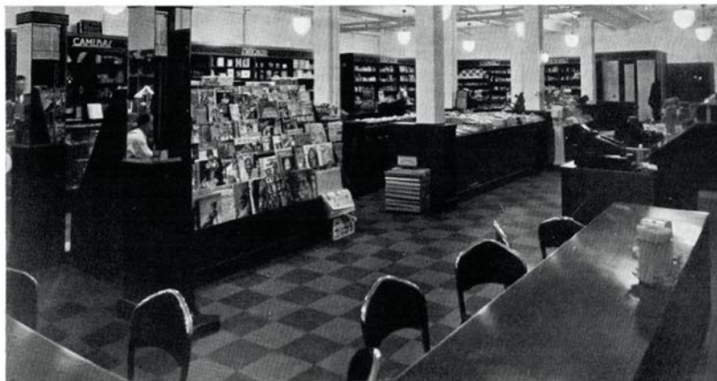
Interior of the new Avenue Store on Second Street. The floor space is 33 by 65, and equipped with every modern convenience.
