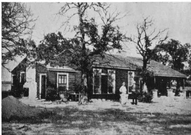
House built entirely of newspaper cores by Mr. P. Lucas, of Dallas, Texas.
