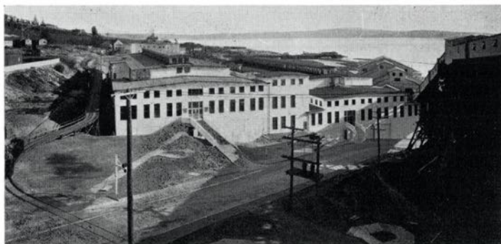
Exterior of No. 7 and 5 and 6 machine rooms as they appear today. The old construction shacks on page 2 have disappeared to give place to the new grinder room shown in the above background.
