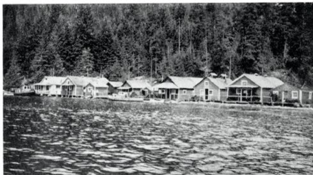
Typical "city on logs." One of the logging camps in the Queen Charlottes. These "cities" are towed by tug from place to place as desired.
