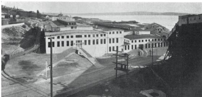
View of No. 7 (left) and 5 and 6 machine-room buildings, taken from the top of the boiler house.
