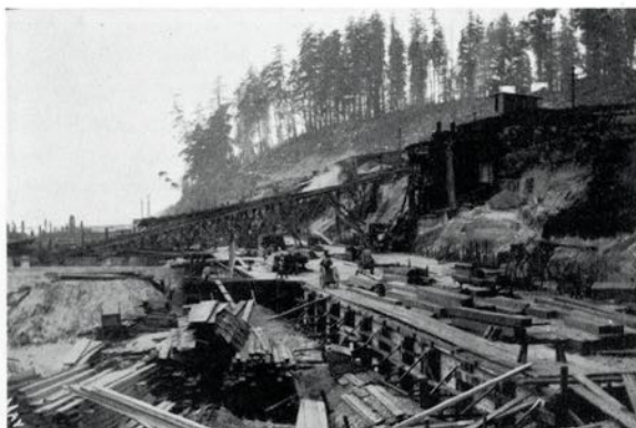
The beginning of mill construction in 1911. Foundations are being laid for the original grinder room and paper storage. Clearing operations in this section were very difficult.
