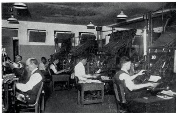
One of the batteries of linotypes that set news in the composing room on the third floor.
