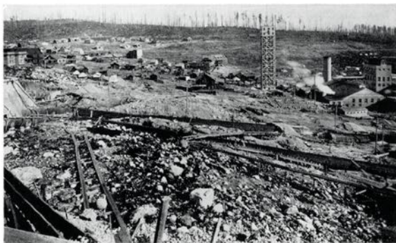
View of the townsite early in 1912. The old acid tower is seen in the course of construction and the original steam plant has just been completed. A few houses in the background show the beginning of townsite construction.
