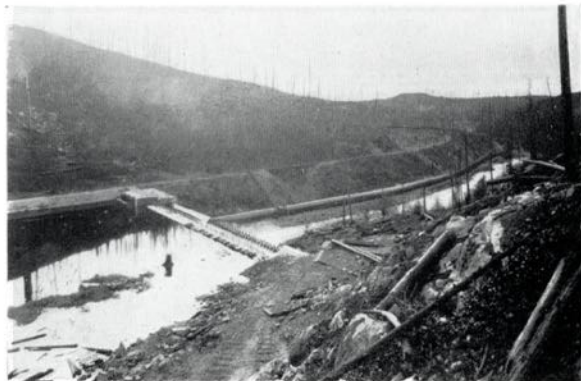
Side view of the temporary log crib dam at Lois, showing the 10-foot temporary wood stave pipe line, running along the old river bank. On the hill, a few hundred yards from this point the big 214-foot flagpole, now in Kew Gardens, London, was fallen.
