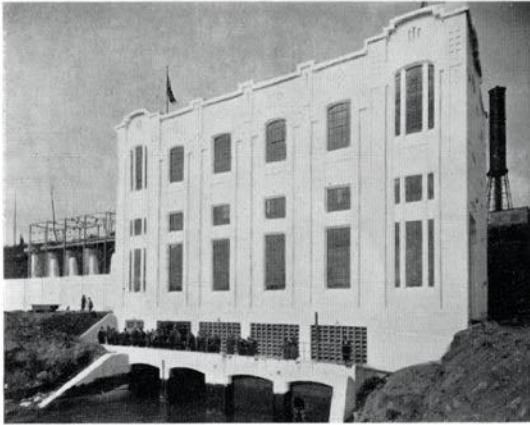
Splendid view of the new Stillwater powerhouse, regarded as one of the best and most artistically designed of its kind on the Pacific Coast.
