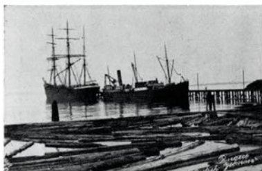
The barque, British Yeoman, bringing in the first load of concrete for plant construction in 1911. The old sailing craft were seldom seen at our dock after this date.
