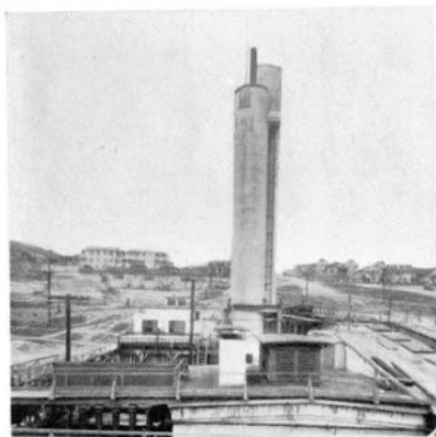
View of the acid tower, where the sulphurous acid is formed by the action of lime rock, sulphur and water. From here, the acid is sent through the pipes to storage tanks and thence to the digesters.
