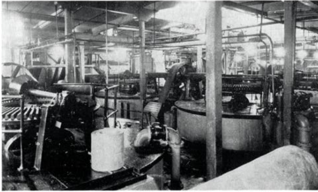
Section of the beater room, showing tanks.
