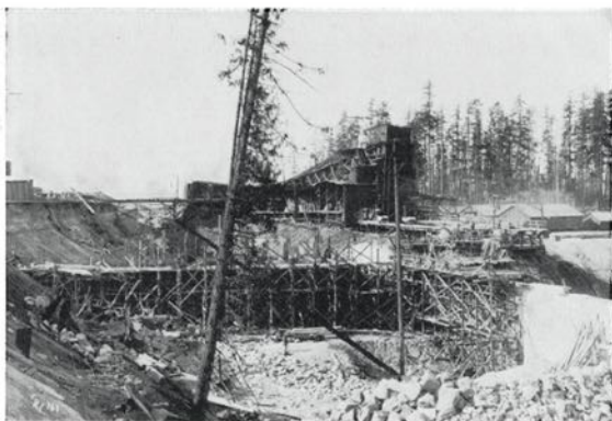
Another view of the dam in 1911 showing the west side under construction. The camp on the right is the Wells Construction Company where the boys spent their evenings before houses were a regular part of the townsite.
