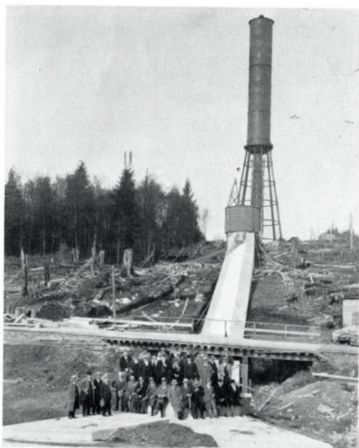
Splendid view of the completed development work at Lois River taken during the recent visit of the safety delegates to Powell River. In the background is the penstock line overtopped by the big 315-foot surge tank. In the foreground, the "wye," with its two 7' 9" branches, may be seen.
