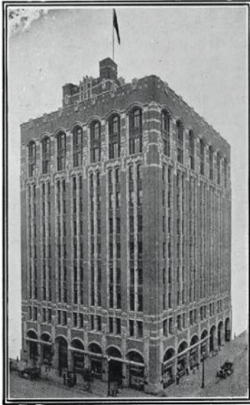
View of the present home of the Calgary Herald, at Calgary, Alberta. The building is a ten-storey fireproof structure, one of the finest newspaper buildings in Canada.
