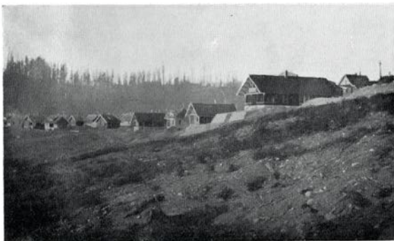
The beginning of townsite construction in 1910-1911. The Directors' house is shown in the foreground, and the beginnings of clearing along Ocean View.
