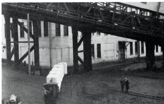
Locie, with her trainload of paper passes underneath the log conveyor, en route to the storage sheds.
