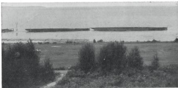
Former United States cruisers are becoming everyday incidents in Powell River. Photo shows the hulls of the former cruisers, U.S.S. Charleston and Huron, now forming a portion of Powell River log defence against the winds of Malaspina Straits.
