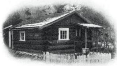
Mr. F. Whicker's log cabin home at Cranberry.
