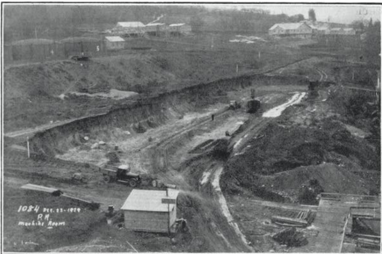
The first beginnings of a new paper machine. Steam shovel at work on excavation for the new machine room, the first unit of which will be ready in 1931.
