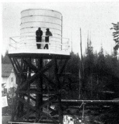
The 5000-gallon tank into which the water is forced from the dam, and from there distributed to the members of the Squatters Creek Water Corporation.
