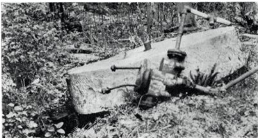
Relics of British Columbia's first paper mill still exist on the old site. Here is one of the beater stones as they appeared recently.
