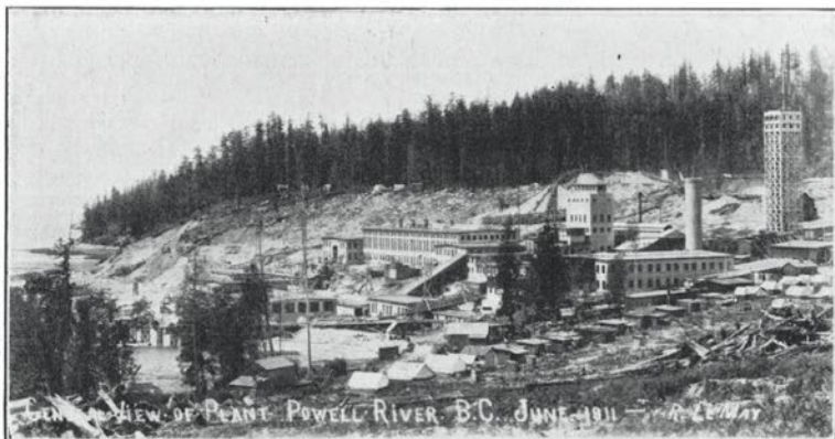
How Powell River looked in June, 1911. The first unit of our plant was nearing completion and ready for the installation of the paper machinery.
