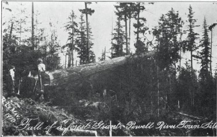
Before there was a townsite. Falling giant timbers during clearing operations, early in 1910.
