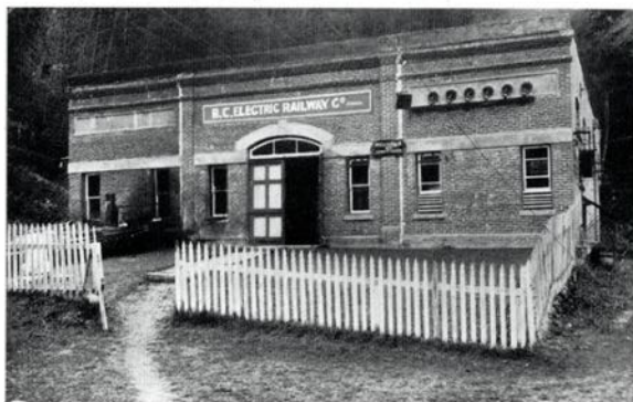
The plant of the B. C. Electric Railway at Gold- stream, Victoria, first hydro devel- opment on the B. C. Coast.
