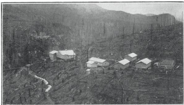
The beginning of construction at Stillwater; the camp above Lois River falls, where work is now proceeding on the new tunnel.
