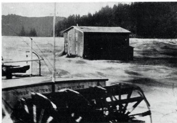
Here is an original picture of the old Station A plant at Oregon City, Oregon, loaned by Mr. Bruce Zumalt, plant superintendent. This was among the first, if not the first, hydro development on the Pacific Coast, installed in 1889.
