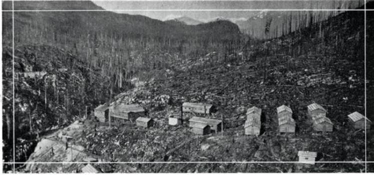
Camp 3, at Lois River, on the bill facing the north portal of the tunnel now under construction. This land was logged many years ago by Brooks-Scanlon-O'Brien.
